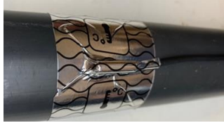
Fig 4 – Temperature Probe Installation
